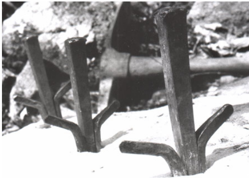
Wedges and shims in place
